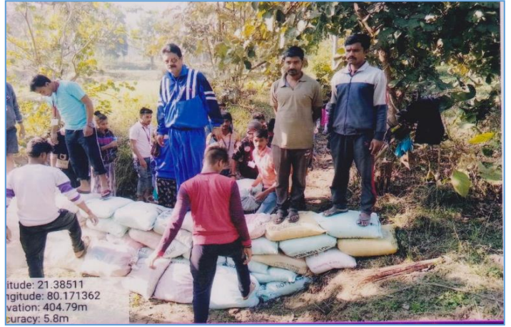
NSS Volunteers constructing the Vanrai Bandhara at Satwa Village
