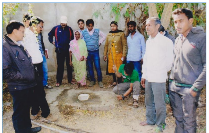
NSS Valunteers constructing toilet in NSS during camp
